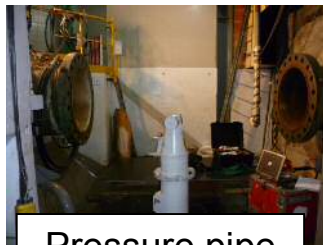
Pressure pipe alignment
